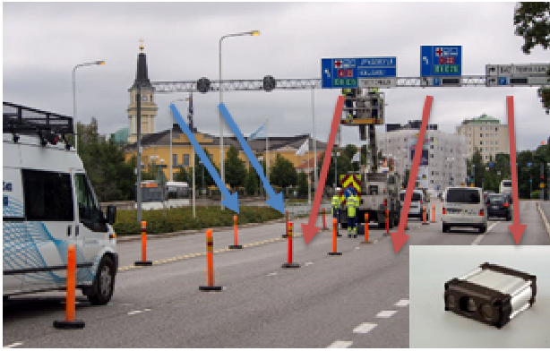
Fig. 1. Installing dual laser measurements sensors and cameras to detect traffic flows, amount of snow, and fleet speed in each lane. A local energy company assists in providing the electricity and connectivity. Companies provide the devices, whereas the data are processed in the companies and research institutes. City of Oulu, 2014.
